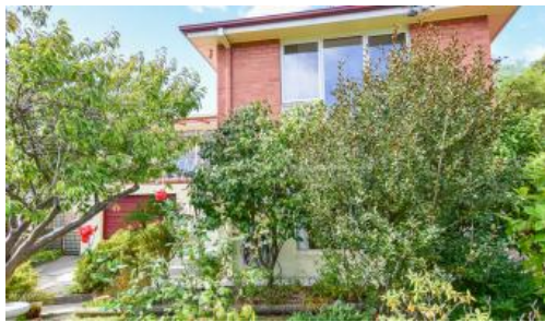
46 Pitt Avenue, Riverside
